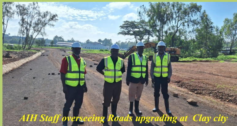
Clay city Roads upgrading
