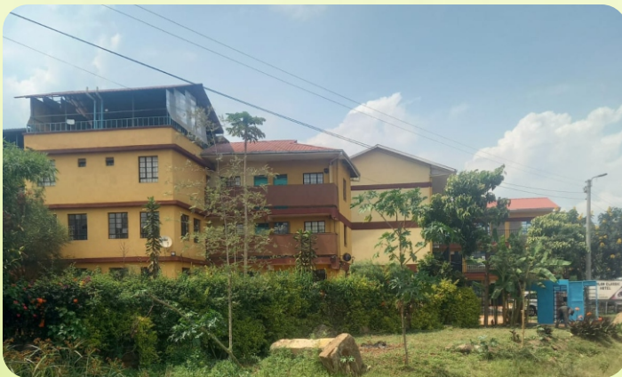
Ongoing Developments by plots owners at Kenyatta Road
