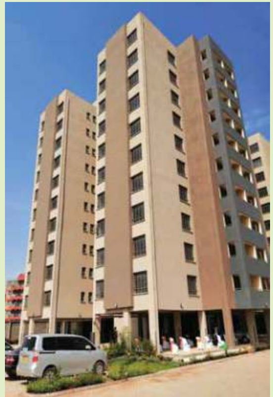
Completed Claycity Apartments Phase one comprising of 80 Units of 3 Bedrooms. Handed over to buyers on 5th June 2020.
