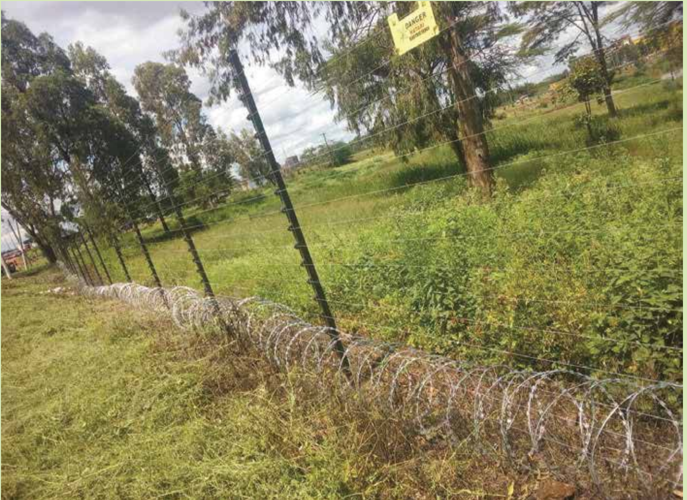
Clayworks Campany Land fenced using electric fence to avoid destruction and not like in the past where hooligans hired by land grabbers used to uproot and damage the fence as shown below.
