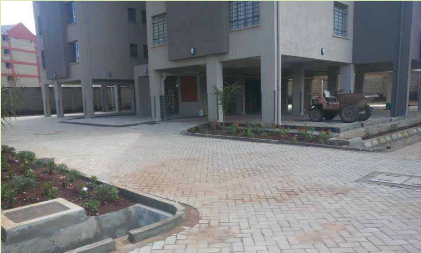
Showing completed landscaping
