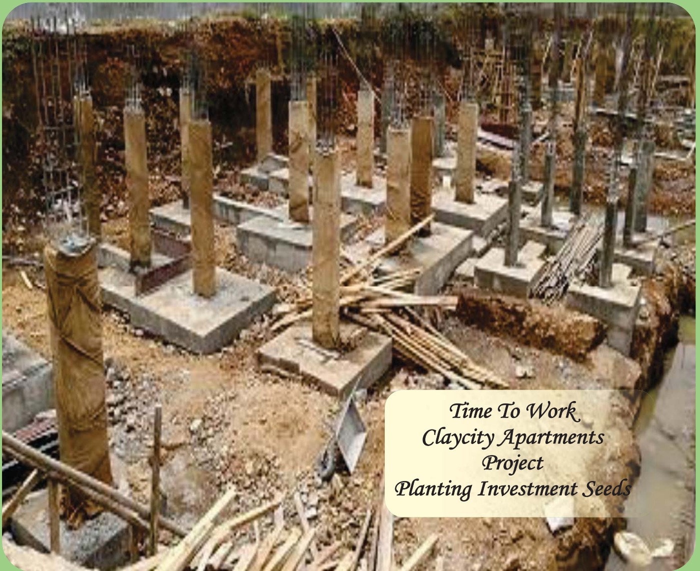
Claycity Apartments Construction work – Foundation Columns
