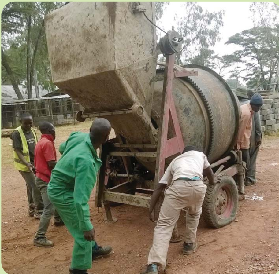
ClayCity Apartments project , Jinsing Ent Co. Ltd workers on site
