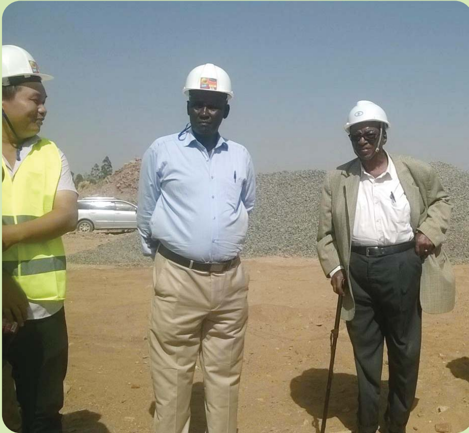
From Right Chairman Hon. E.M. Wamae, GM Mr. Michael Wandegwa and Mr. Wanga of Jinsing Ent Co. Ltd. on inspection tour of Claycity Apartment Construction. Time to work, the Chairman Leading by example.
