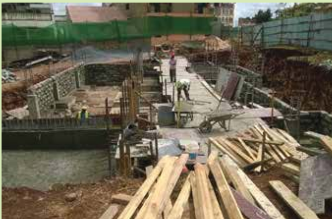
Start of new office block foundation
