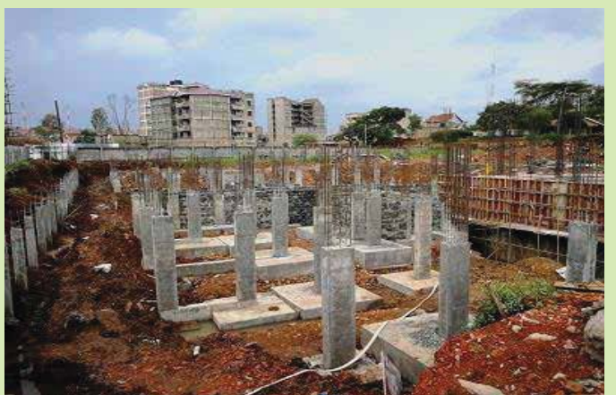
Block A 6 Foundation Columns
