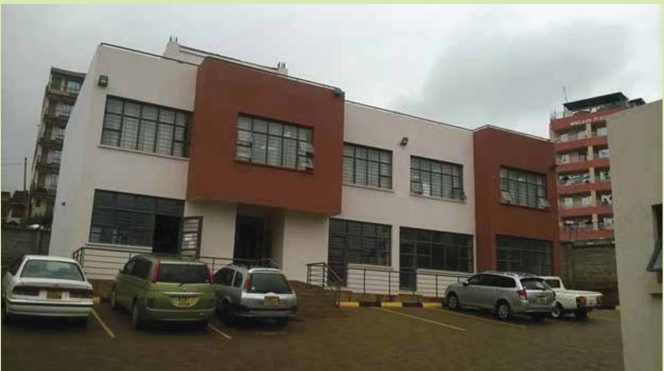
New office Block, hosting AIH Ltd head office in 2018.
